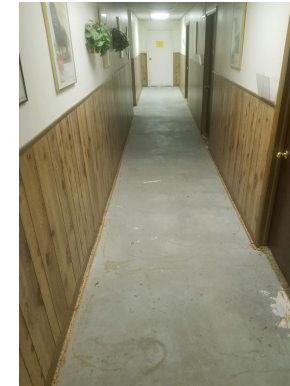
Long Hall In 2 nd Bldg.
