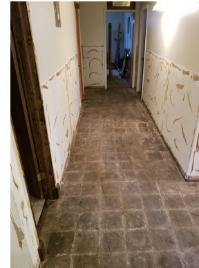
North Hall In 1 st Bldg.
